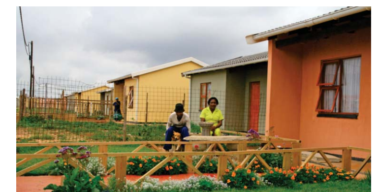
Human Settlement Project in Polokwane
